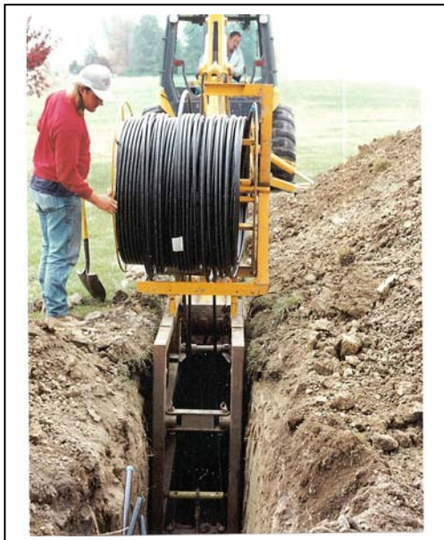
Figure 20 – Installing Horizontal Loop 20
