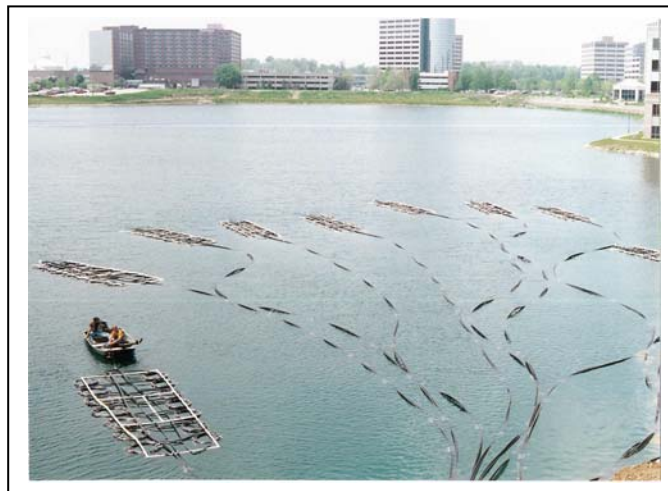
Figure 25 – Installing Pond Loop 22
